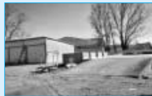
Centre Technique Municipal
